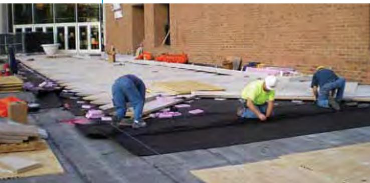
“Our scope of work included demolition of the existing concrete planters and topping slab, down to the structural deck,” Berndt continues.
