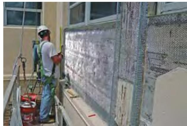
*The scope of the 32 West Gore project increased significantly when Western discovered lath deterioration four inches deep—twice that originally anticipated. Swing-stage work requirements and ongoing tenant/guest access made safety a primary consideration. Both the finished project and Western process earned Orlando Health praise.*
