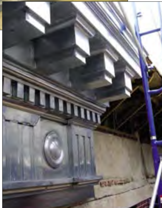
Seventy years of wind and weather had compromised the intricate beauty of 40 Tiemann’s distinctive metal cornices. Craftsmen from Michigan Ornamental fabricated 144 lineal feet of design-enhanced replacements to restore the building’s original elegance.
